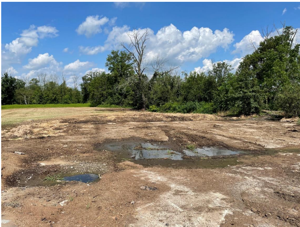
Photo 6 – Concrete storage pad previously used for composting animal remains and processed compost spread on adjacent land with stormwater accumulated on spread material Taken by Jennifer Ramos-Buschmann on 8/17/23, 11:32 AM
