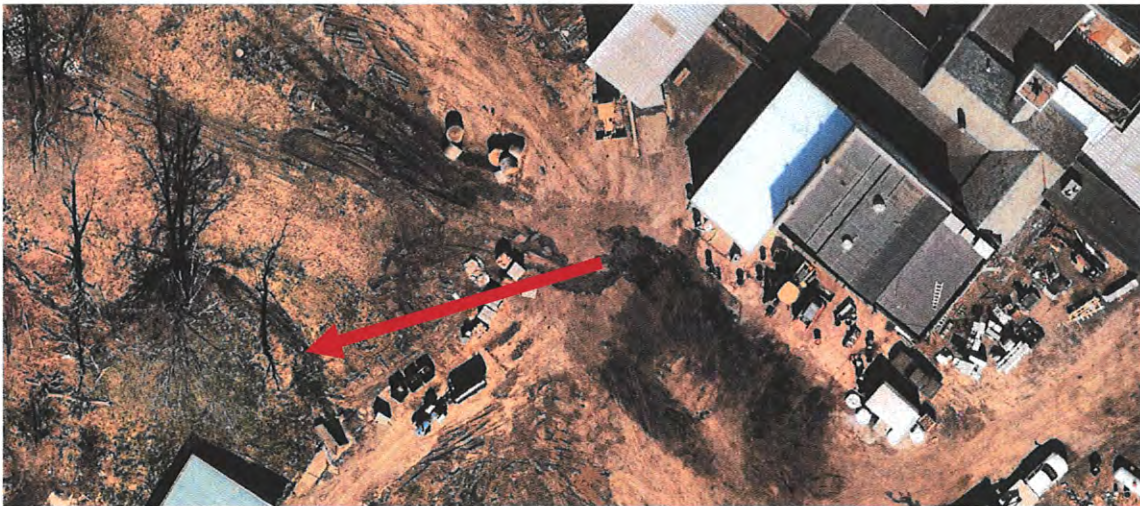
Prevent waste material from entering creek drainage way.
