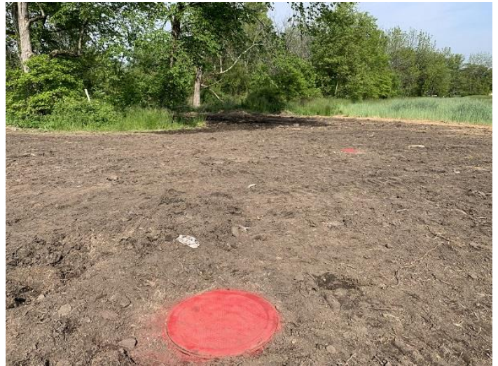
Wastewater system manhole. Seep discharge point is at rear
