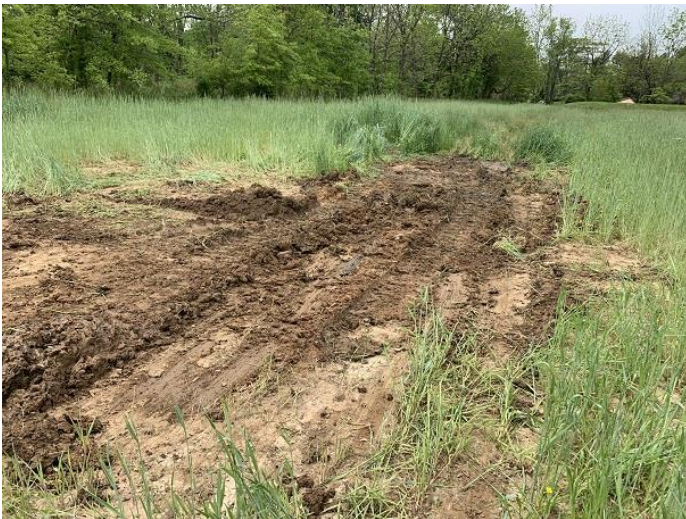
Excavation of a field seep
